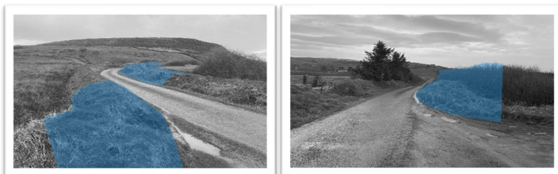
Figure 2.4 – Visibility Splays Partially Obscured in Both Directions at Location 6 Forestry Access
