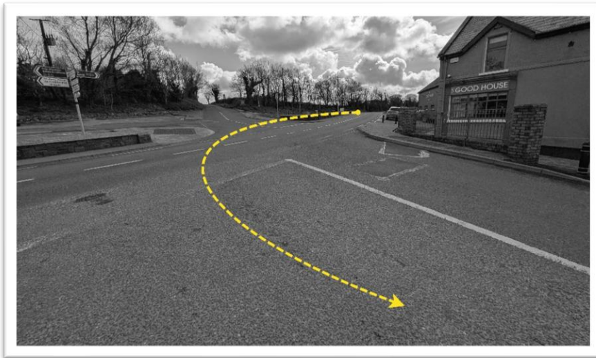
Figure 2.1 – Image of Location 1, N85 / R460 Junction for Record Purposes Only
